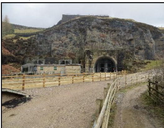
The Woodhead portals today. The old single bore tunnels are on the left and the new tunnel, with the cable ducts, is on the right. photo:Paul White
